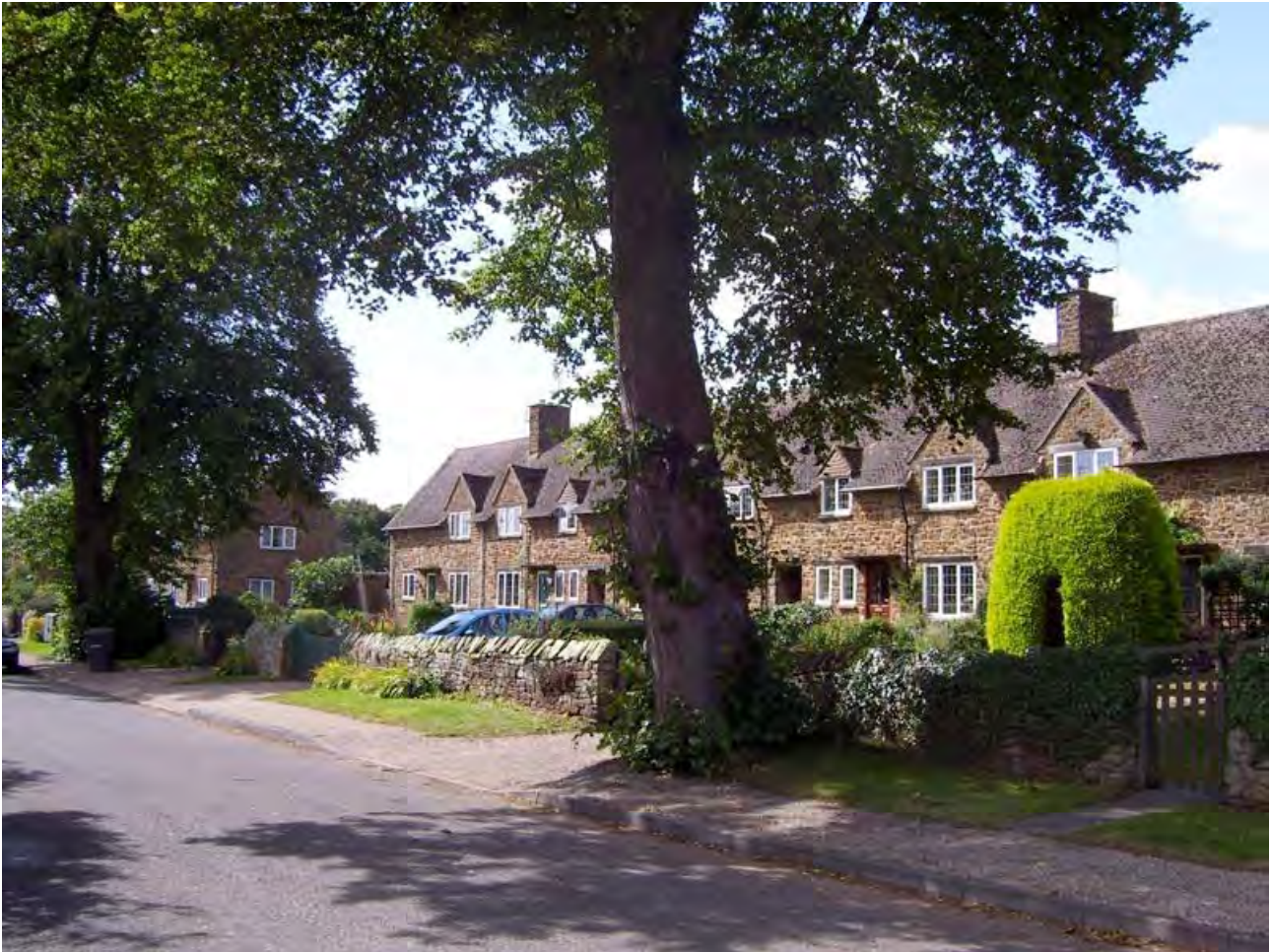
Lime Avenue's prize-winning council houses
