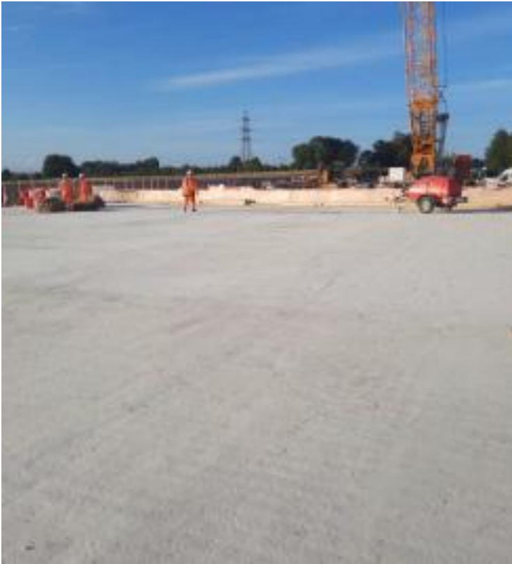
Concrete deck complete
